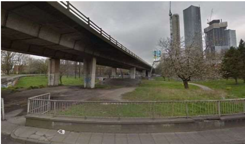
Mancunian Way bridge
