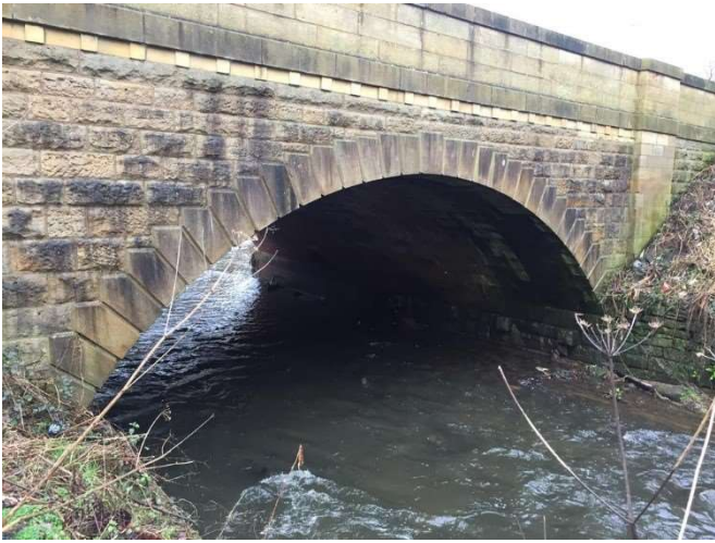
Heaton Park Road Bridge, River Irk;
